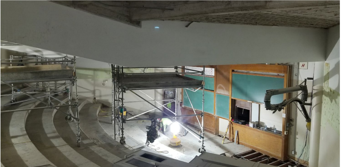
Gilbert 124 in mid-demolition
