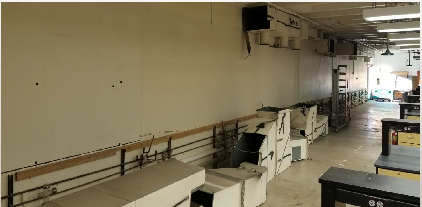
GBAD 209 with the Fume Hoods removed
